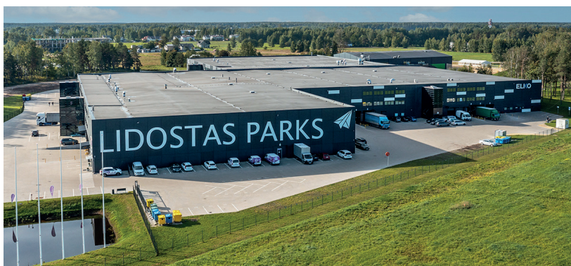
Lidostas Parks, Riga, Latvia. Modern warehouse, production and office complex.
