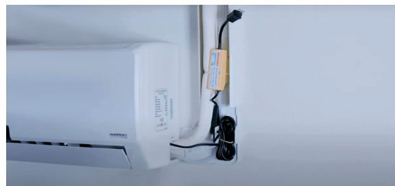
Solution with an externally incorporated condensate pump.
